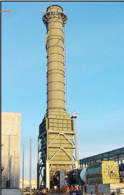
One of three 215 ft tall exhaust stacks installed at an 880 MW power plant in Ontario
