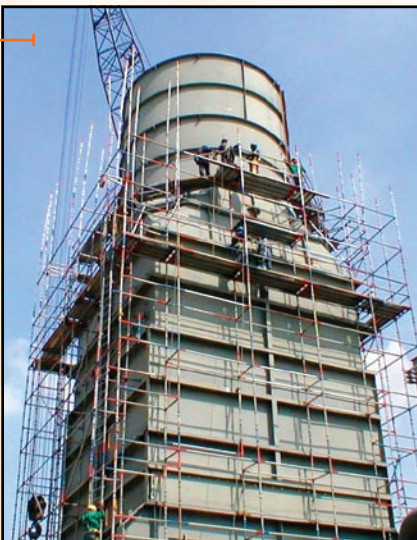
Exhaust system installation for a Siemens 501FD turbine in Venezuela
