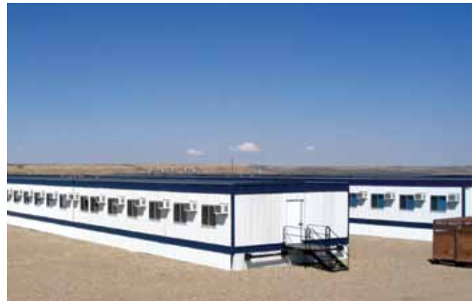
Nabors Drilling, 154 Person Construction Camp, Wamsutter, Wyoming
