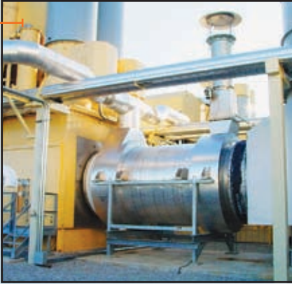
The ATCO/Higgott-Kane Anti-icing System
