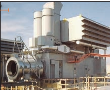
Installation of the exhaust duct heat exchanger
